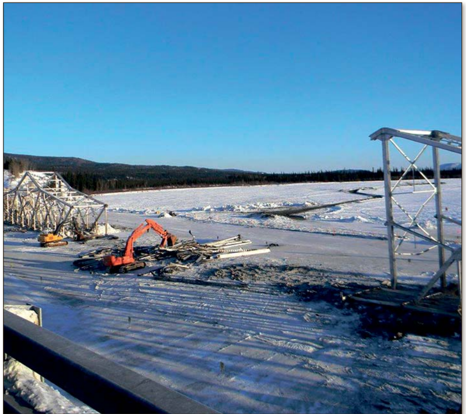
PHOTOS: COURTESY OF ALASKA DEMOLITION LLC
