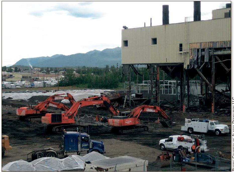
Only a small section of the foundation remains of the Elmendorf coal-fired power plant following demolition by four Alaska Demolition excavator operators in 2007.
